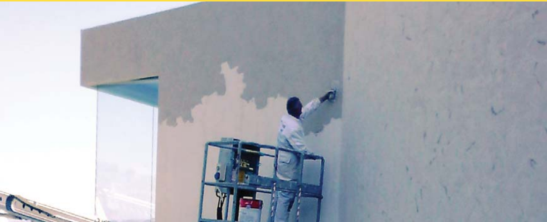
Insulating shaving finish
