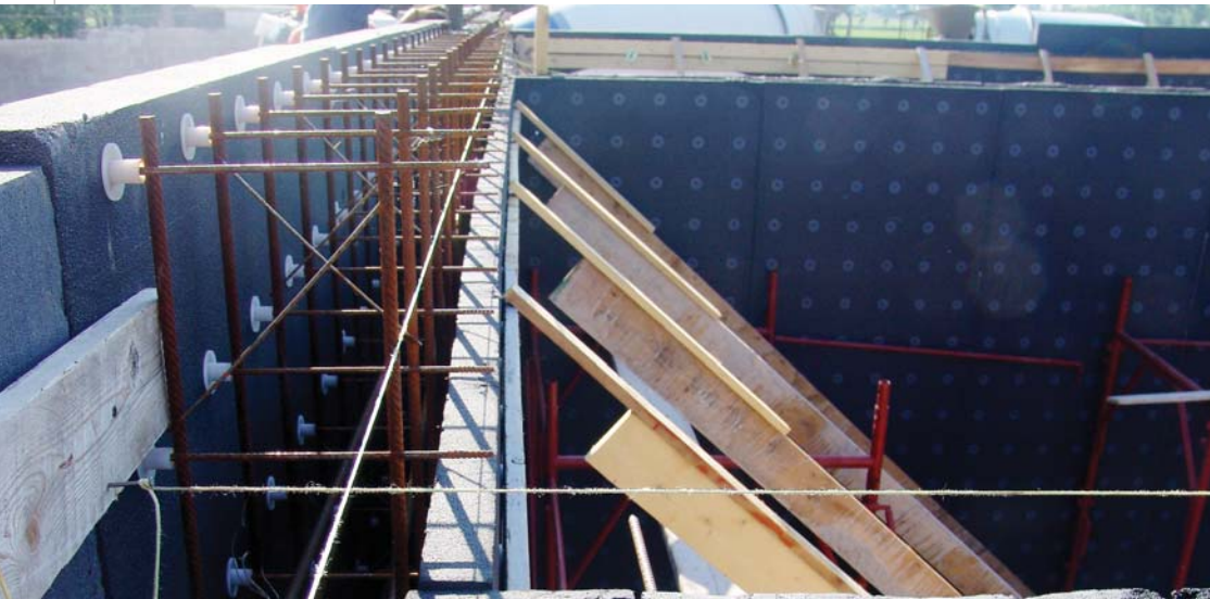
Detail of the rib for floor grid
