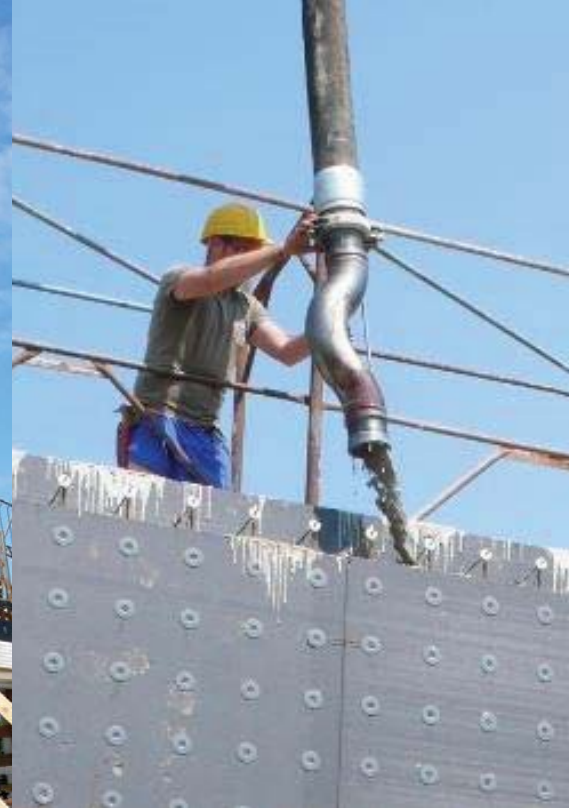
Casting with pump
