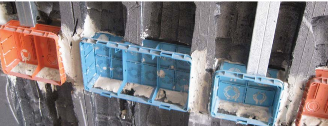
Installations, ducts on the Wall Plastbau® 3 internal panel
