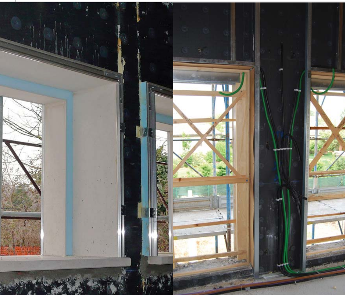
Prefab sub-frame to be mounted before casting
