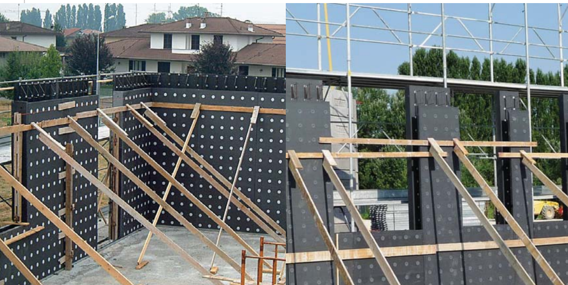
Wall Plastbau® 3 elements put close to one another and plumb, by means of diagonal struts joined by a continuous band -nailed on panel PB3 Plugs
