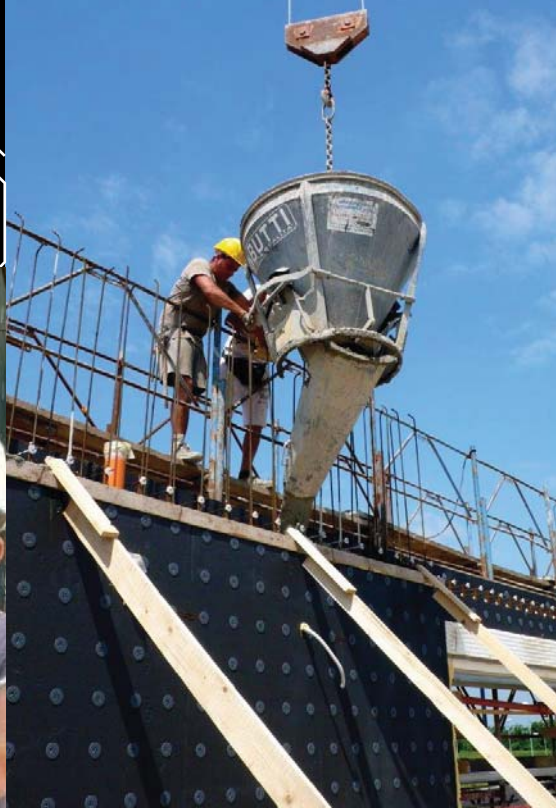
Casting with bucket
