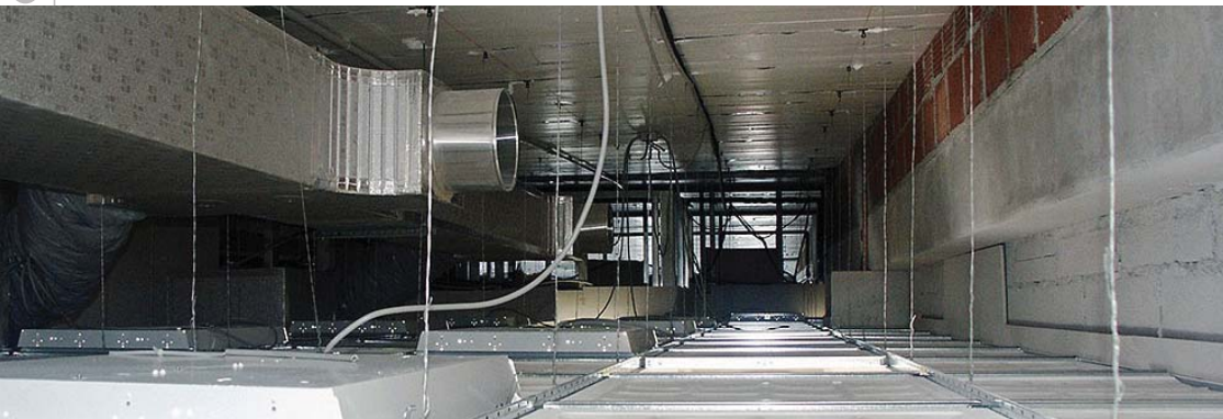
Lowered and dropped false ceiling
